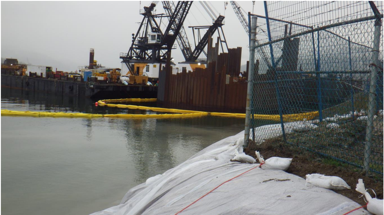
Photo 3. Turbid water being contained by turbidity curtain.
