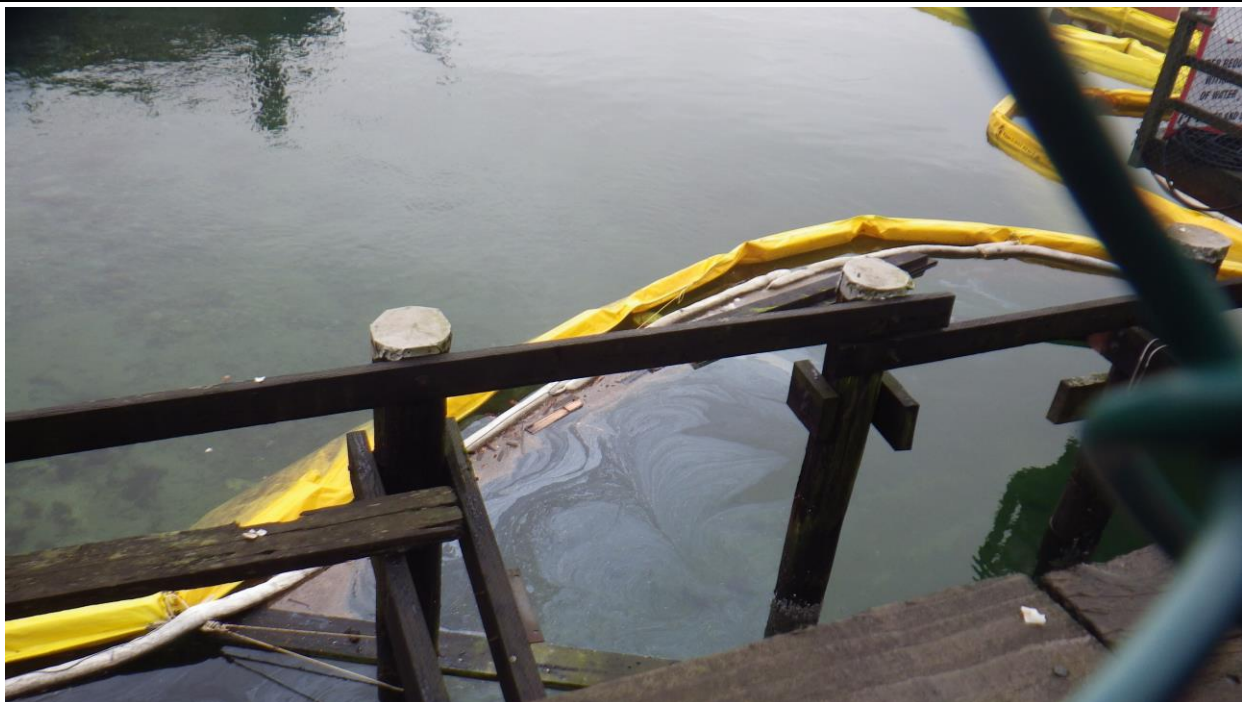
Photo 2. Yellow turbidity curtain and sorbent boom containing saw dust, wood debris, and creosote released during demolition of the utility dock. Any remaining debris is skimmed off the surface of the water at the end of each day.
